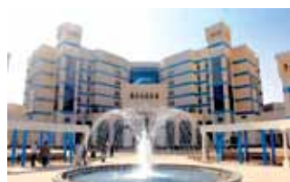
The new Al Wakrah Hospital
